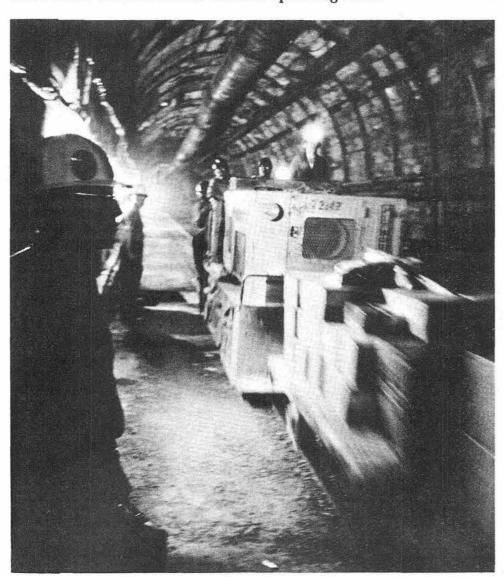
N-TUNNEL EXPRESS carries people and material to experiments located mile-and-a-half down tunnel. Tunnel is actually complex of two main tunnels with innumerable drifts and alcoves. More than ten nuclear shots have been staged here
